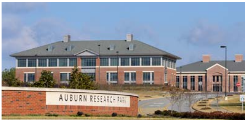
Buildings I and II – Auburn Research Park
